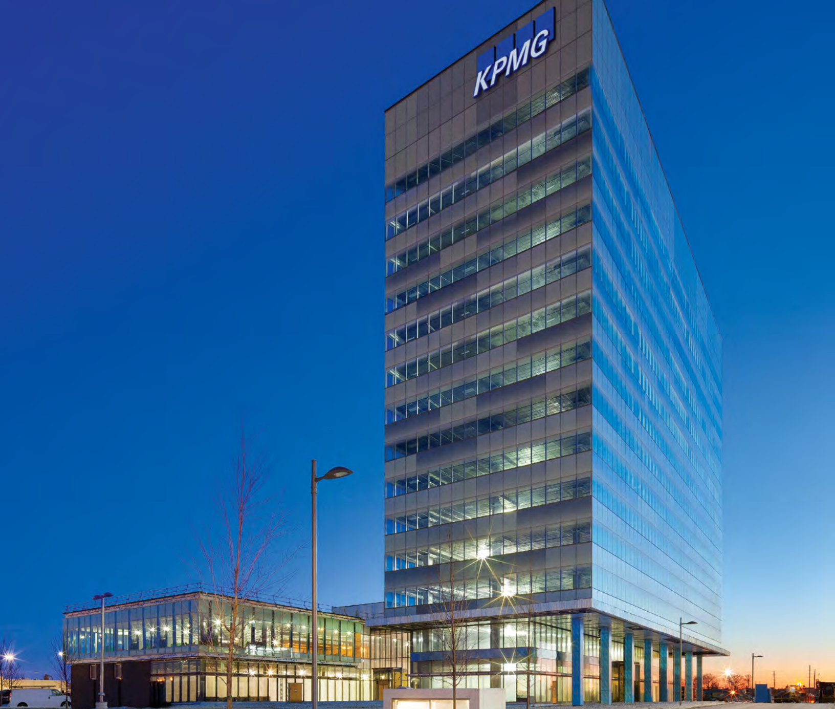
KPMG Tower, VMC, Under Construction, Vaughan, ON
