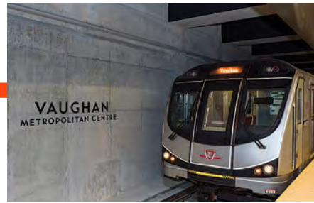
VMC Subway Station
