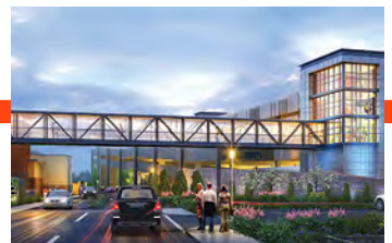
Toronto Premium Outlets Expansion – Multi-level Parking and Pedestrian Bridge
