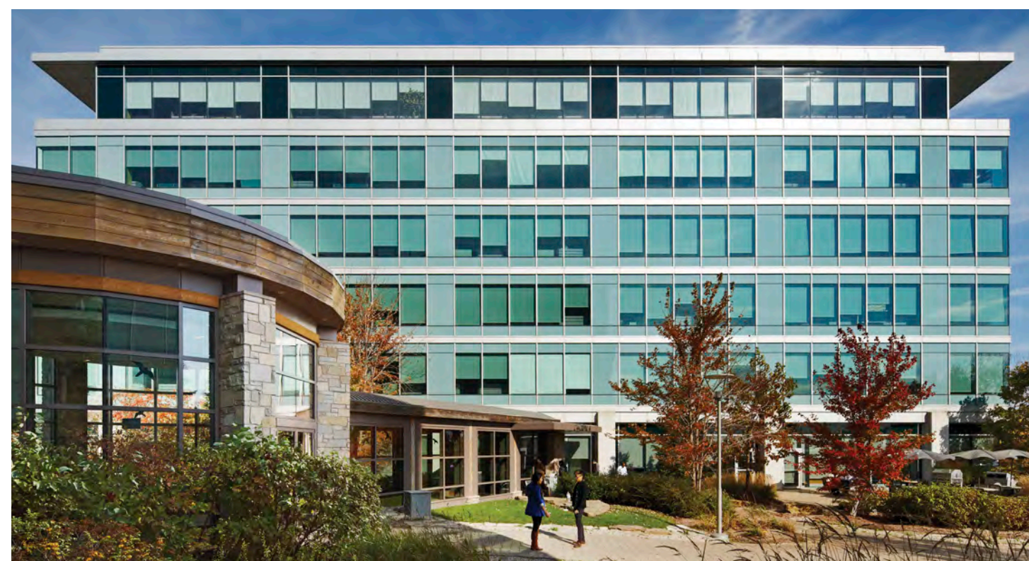
CREEKSIDE CORPORATE CENTRE TORONTO, ON
